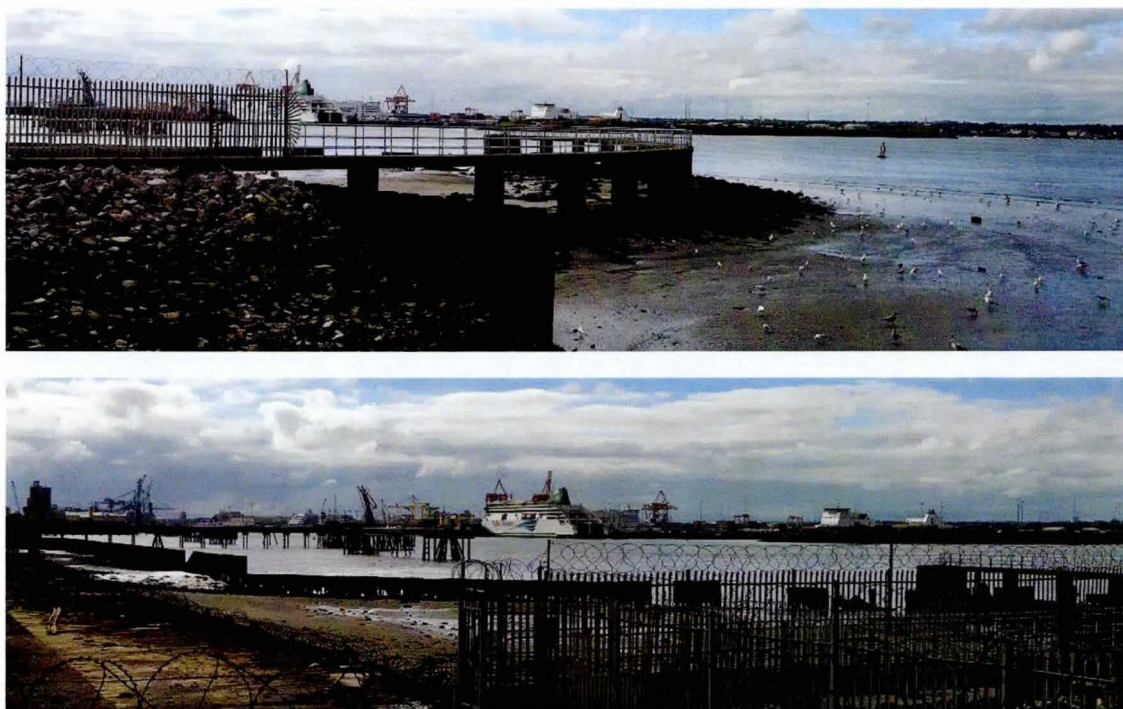
Figure 5.18 Photographs of the Ringsend WwTP outfall location during low tide on 2 nd of August 2016. Top image shows the weir and walkway (section D of Figure 5.17). Lower image shows broken and damaged sheet piles along the back section of the existing weir (Section B and C of Figure 5.17).
