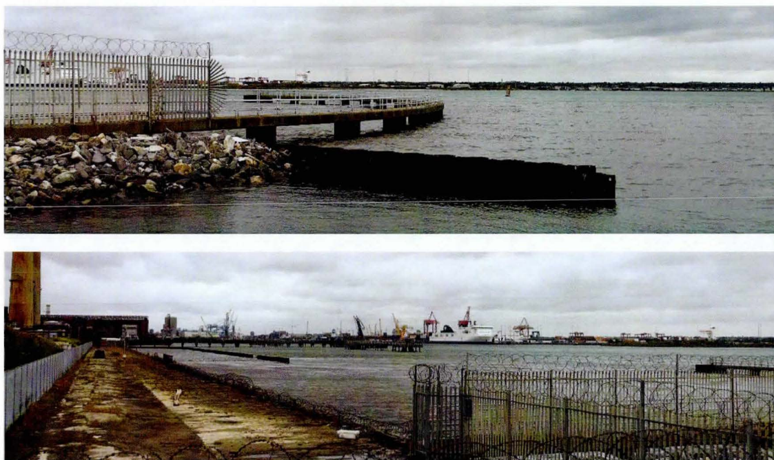
Figure 5.19 Photographs of the Ringsend WwTP outfall location during high tide on 3 rd of August 2016. Top image shows the weir and walkway (section D of Figure 5.17). Lower image shows water flowing into the Lower Liffey over the damaged sheet piles along the back section of the existing weir (Section B and C of Figure 5.17).
